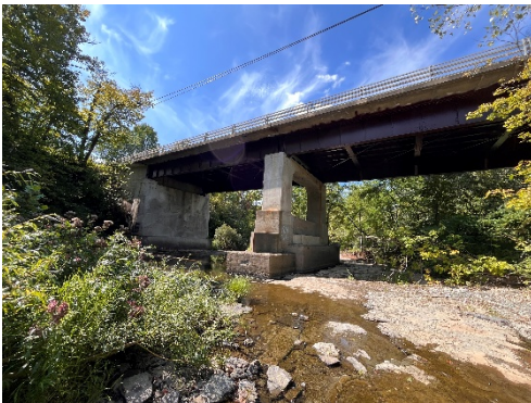
Existing Photo. East elevation of bridge.
