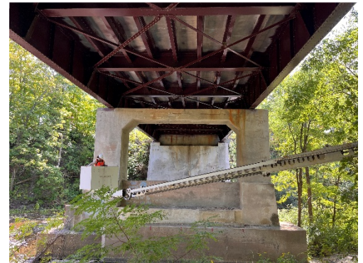
Existing Photo. Taken under the bridge on the north end looking south.
